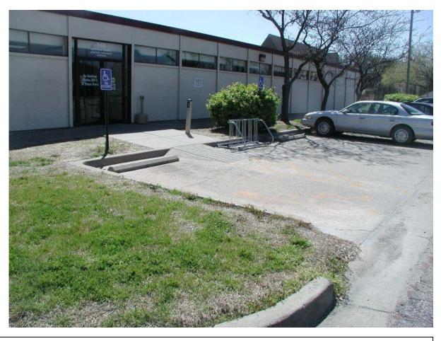
Non-compliant ramp, access aisles, sidewalks, and door landing. Bicycle rack is located in an access aisle.
