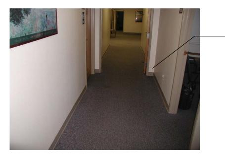
Insufficient maneuvering space, doors must remain open at all times.
