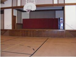
**EXISTING CONDITION:** A stage exists in the multi-purpose room. According to ADAAG, an accessible route shall connect stages, arena floors, dressing rooms, locker rooms, and other spaces used by performers. An accessible route cannot include steps.
