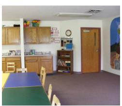
**EXISTING CONDITION:** Doorways to classrooms do not provide appropriate maneuvering space at door. ADAAG requires at least 12-inches to the latch push side of doors when doors have both a closer and a latch per ADAAG Figure 25.
