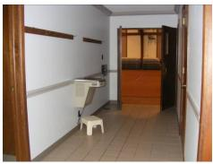
**EXISTING CONDITION:** Drinking fountain in hallway by kitchen is a protruding object that is not **detectable by cane.** Objects that project more than 4" from the wall, 27" above the floor and less than 80" above the floor are not cane detectable.
