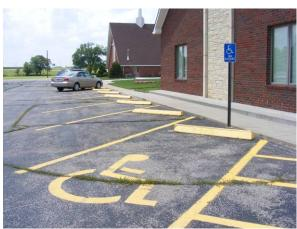
**EXISTING CONDITION:** One van accessible parking space exists to serve the COMCARE program (located near the COMCARE entrance). The slopes, dimensions, and signage comply with ADAAG
