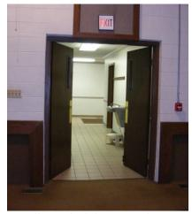
**EXISTING CONDITION:** Entrance doors (to multi-purpose room) provide less that 32" clear opening (each door is 2'-6"). ADAAG requires double leaf doorways to have at least one leaf that provides a clear 32" opening. Doors, leading to accessible facilities, are required to have a minimum clear opening of at least 32-inches measured with the door open 90-degrees.
