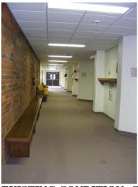
EXISTING CONDITION: Coat racks at hallway by classrooms are located at 48-1/2" to the lowest hook. This complies with current ADAAG, but may be too high at 53" once the New ADAAG is adopted. Where coat racks or hooks are provided, at least one must comply with reach ranges defined by ADAAG 4.2.5 or 4.2.6. The New ADAAG further limits this to a 48" maximum height. (ADAAG 4.25.3, 4.2.5, 4.2.6, & New ADAAG 308)
