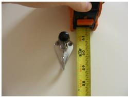
EXISTING CONDITION: Coat hooks in accessible restroom stalls (at Men's and Women's Restrooms) are located too high at 61". Where coat hooks are provided, at least one must comply with reach ranges defined by ADAAG 4.2.5 or 4.2.6. The New ADAAG further limits this to a 48" maximum height. (ADAAG 4.25.3, 4.2.5, 4.2.6, & New ADAAG 308)
