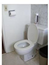
4. Restroom is totally inaccessible due to numerous inconsistencies. Inconsistencies include, but are not limited to, insufficient maneuvering and fixture clearances, inappropriate maneuvering space at entrance doors, no knee space at lavatory, inappropriate lavatory faucet controls, incompliant shower, flush valve controls located on narrow side, no grab bars at water closets or
