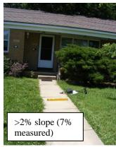
**EXISTING CONDITION:** Abrupt changes in level and steep cross slopes exists on the path of travel (sidewalk) leading to the apartments and the office. According to ADAAG, changes in level up to 1/4 in (6 mm) may be vertical and without edge treatment (see Fig. 7(c)). Changes in level between 1/4 in and 1/2 in (6 mm and 13 mm) shall be beveled with a slope no greater than 1:2 (see Fig. 7(d)). According to ADAAG, nowhere shall the cross slope of an accessible route exceed 1:50 (2%).
