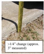
EXISTING CONDITION: No accessible route exists connecting the parking lot with the route (sidewalk) to the office and apartments due to an abrupt change in level (curb) of approximately 3". According to ADAAG, changes in level up to 1/4 in (6 mm) may be vertical and without edge treatment (see Fig. 7(c)). Changes in level between 1/4 in and 1/2 in (6 mm and 13 mm) shall be beveled with a slope no greater than 1:2 (see Fig. 7(d)).
