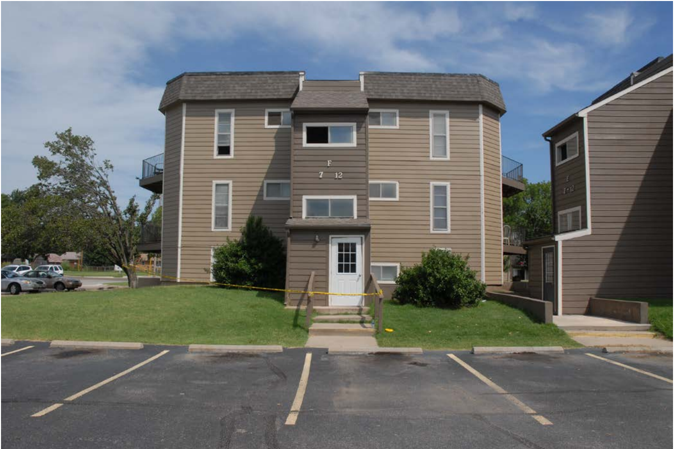
Outside of incident location
