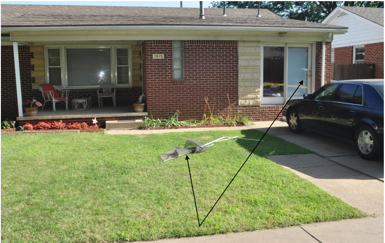
Torn screen and frame from front door of 7815 E. Clay
