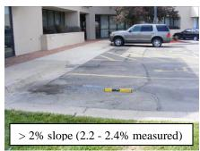
**EXISTING CONDITION:** All accessible spaces and the access aisle slope away from the building with slopes exceeding 2% for the portion of the parking space closest to the building. (ADAAG 4.6.3, 4.6.6)
