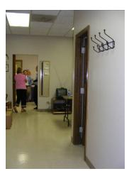
**EXISTING CONDITION:** Coat rack is located too high at 5'-7" and creates a protruding object by projecting 4-3/4" from the wall.
