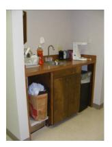
**EXISTING CONDITION:** Sink is too high, does not provide appropriate knee clearance due to cabinets underneath, and has round knob for faucet controls.
