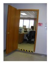
It should also be mentioned that doors at the same location as a step (with no landing), create a safety hazard and generally are not allowed by the building code.
