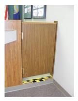
It should also be mentioned that doors (or gates) at the same location as a step (with no landing), create a safety hazard and generally are not allowed by the building code.
