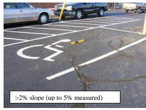
EXISTING CONDITION: The surfaces of designated accessible parking spaces and access aisles east of main entrance are not accessible due to cracked asphalt and slopes beyond 2% (as identified in Kent Johnson's November 2006 report).
