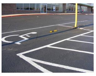
**EXISTING CONDITION:** Accessible parking spaces west of main entrance exceed allowable slope as shown above. Existing slopes measured over 4%.
