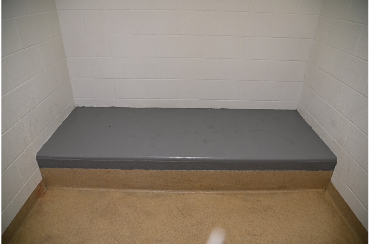
The interior of holding room #1.
