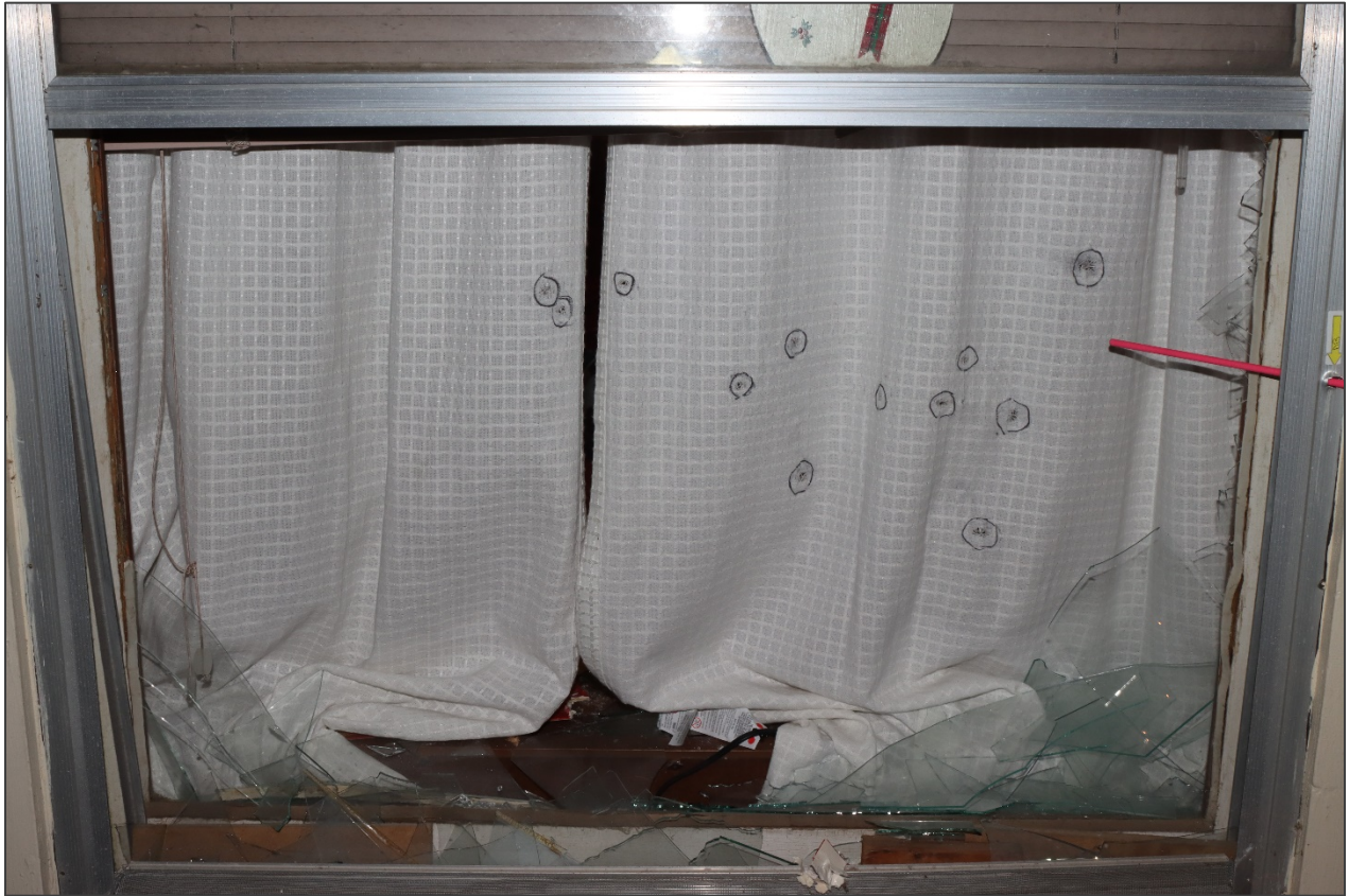
Side window (apparent point of entry) with bullet holes in curtain.
