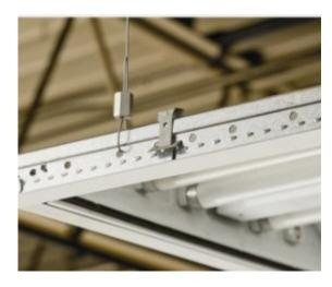
Lighting fixtures in a suspended ceiling system are required to be "positively attached" to prevent fragmenting and dislodging in a seismic event and causing possible harm and injury to building occupants.
