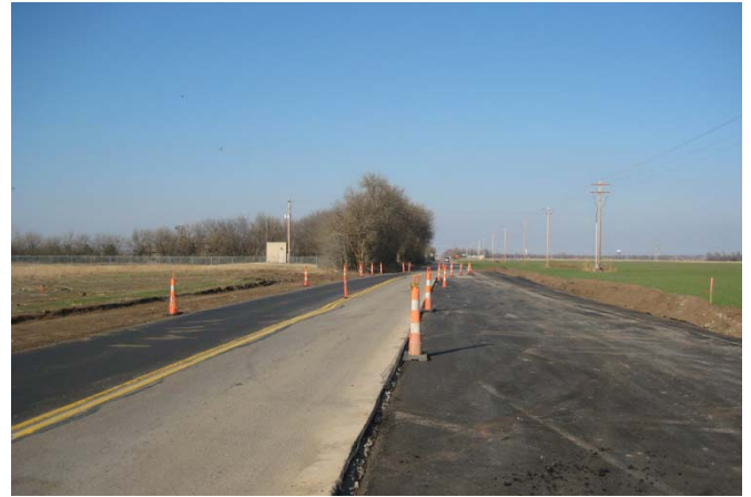
Reconditioning of 119 Street west in progress
