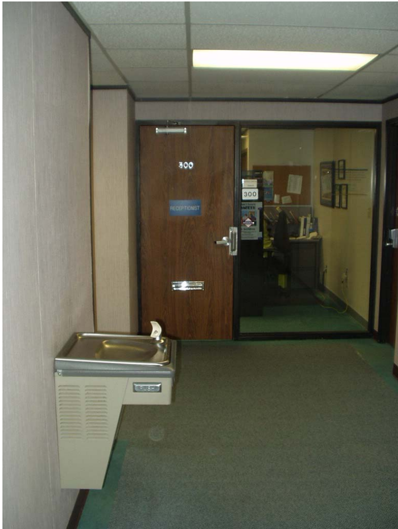
Third Floor Fountain
