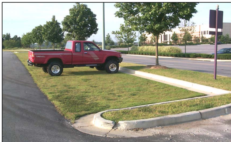
Grass Paver Surface Used for Parking
