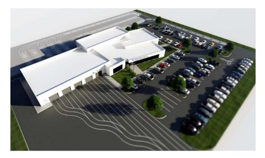
The schematic design has three distinct areas. The first area is vehicle storage and access, with five (5) bays, three (3) vehicles deep, allowing a potential to treat 15 vehicles at once – consisting of a total of 9,571 square feet. The second area is warehouse storage of 4,660 square feet. The third area houses administrative functions and the EOC with 12,486 square feet of space. The proposed building has a total of 26,717 square feet.
