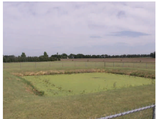
Example of an improperly maintained lagoon: plants have begun growing inside the lagoon.
