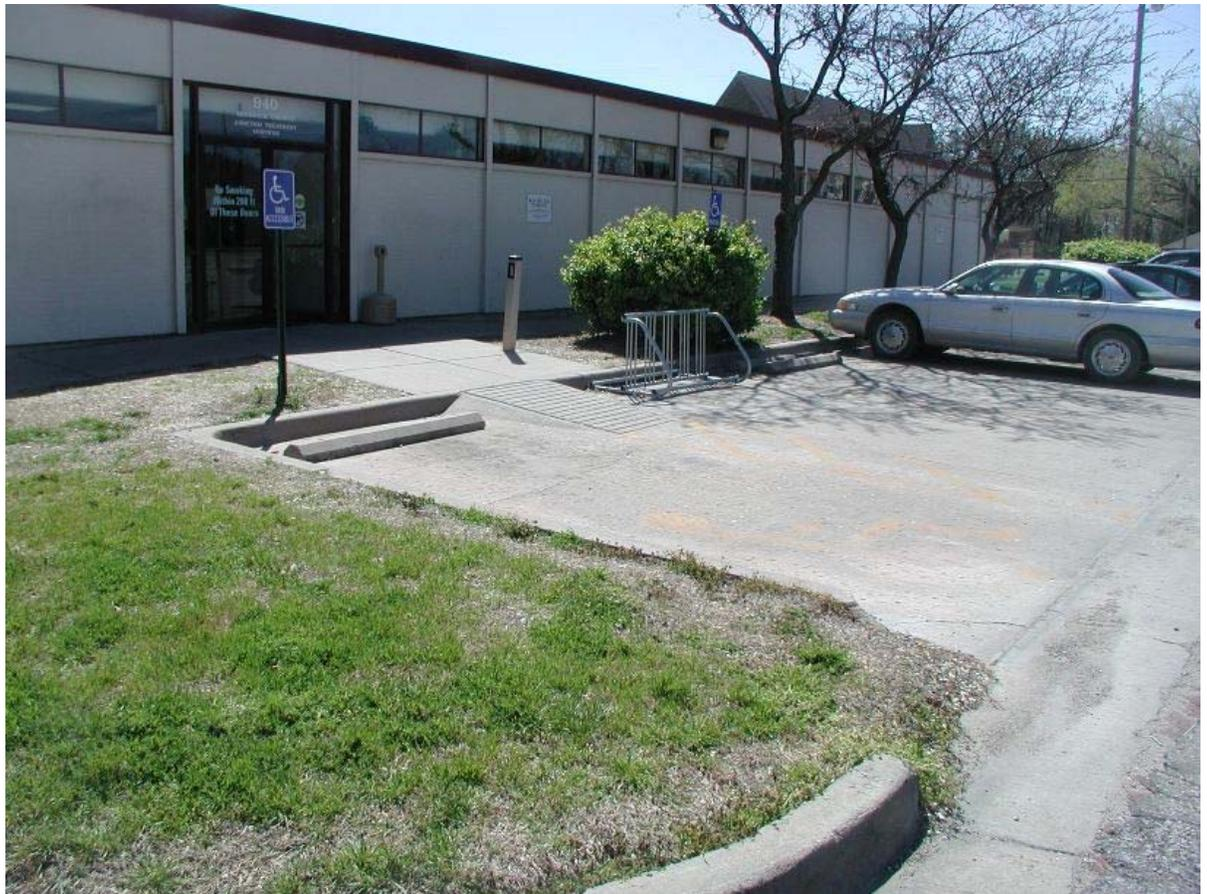
Non-compliant ramp, access aisles, sidewalks, and door landing. Bicycle rack is located in an access aisle.
