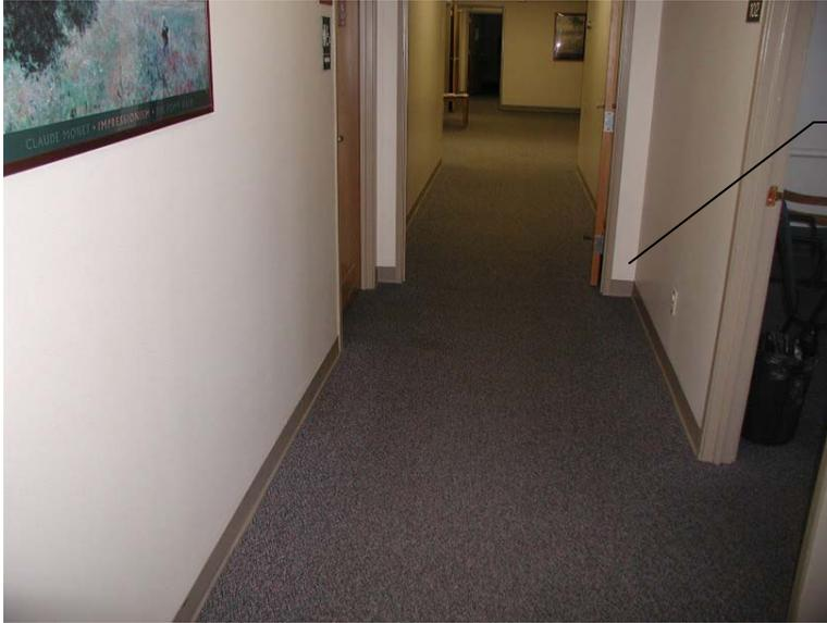
Insufficient maneuvering space, doors must remain open at all times.
