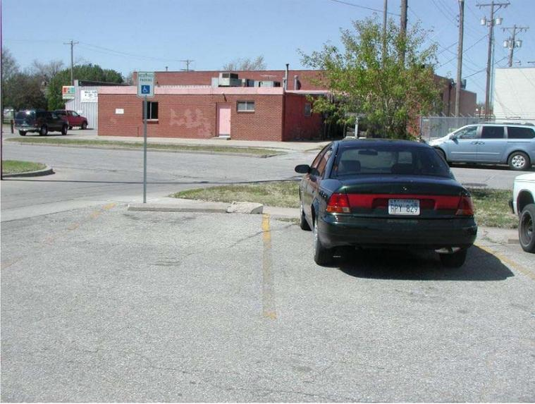
No access aisle. Parking space is required to be 132" wide with a 60" Access aisle.
