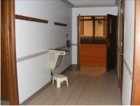
**EXISTING CONDITION:** Drinking fountain in hallway by kitchen is a protruding object that is not detectable by cane. Objects that project more than 4" from the wall, 27" above the floor and less than 80" above the floor are not cane detectable.
