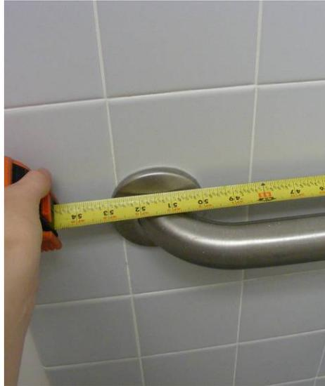
**EXISTING CONDITION:** The side grab bars at the Men’s and Women’s Restrooms comply with the current ADAAG (at 52”); however, the new ADAAG increases the side grab bar dimension from the back stall wall from 52” to 54” minimum. Per the new ADAAG, the side wall grab bar shall be 42 inches (1065 mm) long minimum, located 12 inches (305 mm) maximum from the rear wall and extending 54 inches (1370 mm) minimum from the rear wall.
