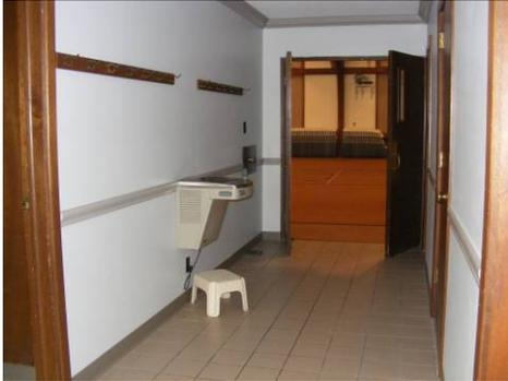
**EXISTING CONDITION: Coat racks at hallway by kitchen are located too high at 64”.**
