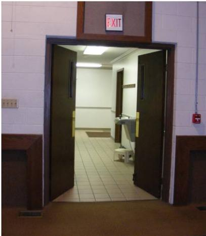
**EXISTING CONDITION: Entrance doors (to multi-purpose room) provide less than 32” clear opening (each door is 2’-6”).** ADAAG requires double leaf doorways to have at least one leaf that provides a clear 32” opening. Doors, leading to accessible facilities, are required to have a minimum clear opening of at least 32-inches measured with the door open 90-degrees.
