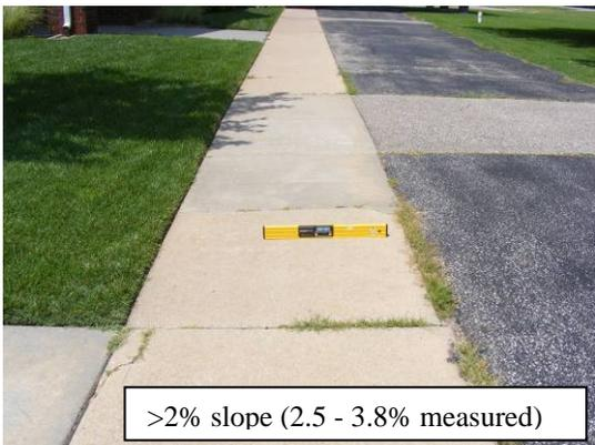
**EXISTING CONDITION:** A small portion of the sidewalk (on route from parking to building) is not accessible due to cross slopes over 2%. According to ADAAG, nowhere shall the cross slope of an accessible route exceed 1:50 (2%).
