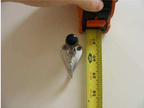
**EXISTING CONDITION:** Coat hooks in accessible restroom stalls (at Men’s and Women’s Restrooms) are located too high at 61”. Where coat hooks are provided, at least one must comply with reach ranges defined by ADAAG 4.2.5 or 4.2.6. The New ADAAG further limits this to a 48” maximum height. (ADAAG 4.25.3, 4.2.5, 4.2.6, & New ADAAG 308)
