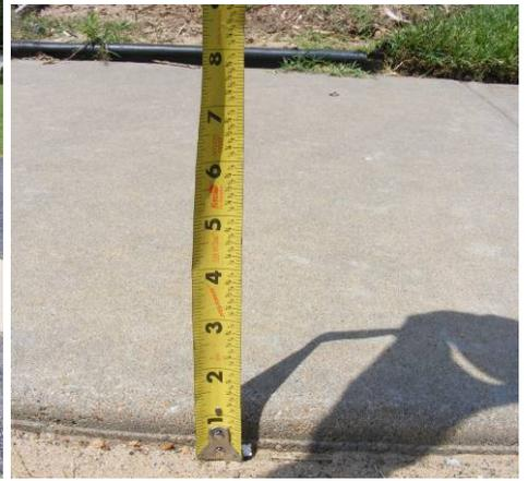
**EXISTING CONDITION:** An abrupt change in level of 1/2" - 3/4" exists on the path of travel from the access aisle to the sidewalk. This occurs where the sidewalk meets the asphalt paving. According to ADAAG, changes in level up to 1/4 in (6 mm) may be vertical and without edge treatment (see Fig. 7(c)). Changes in level between 1/4 in and 1/2 in (6 mm and 13 mm) shall be beveled with a slope no greater than 1:2 (see Fig. 7(d)).
