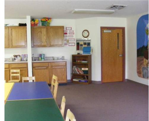
**EXISTING CONDITION:** Doorways to classrooms do not provide appropriate maneuvering space at door. ADAAG requires at least 12-inches to the latch push side of doors when doors have both a closer and a latch per ADAAG Figure 25.
