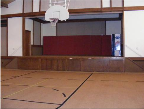
**EXISTING CONDITION:** A stage exists in the multi-purpose room. According to ADAAG, an accessible route shall connect stages, arena floors, dressing rooms, locker rooms, and other spaces used by performers. An accessible route cannot include steps.
