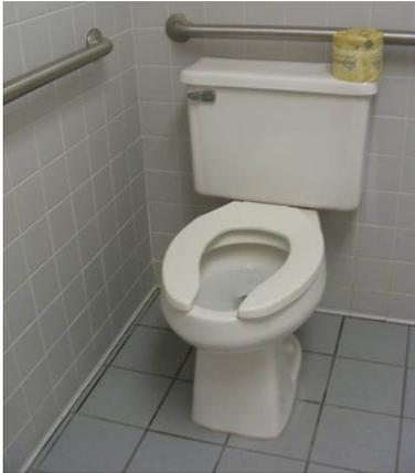
**EXISTING CONDITION:** The flush control for the Men's Restroom water closet is located on the wall side. ADAAG requires that controls for flush valves be mounted on the wide side of toilet areas no more than 44 in above the floor.
