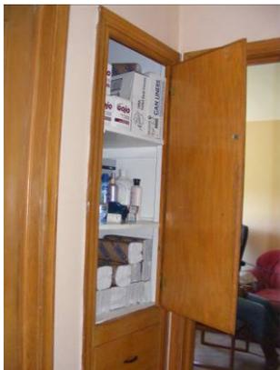
3. **Closet rods are located too high at 64-1/2". Closet door opening hardware is too high at 58".** Storage in accessible spaces in dwelling units, including cabinets, shelves, closets, and drawers, shall comply with 4.25. Accessible storage spaces shall be within at least one of the reach ranges specified in 4.2.5 and 4.2.6.
