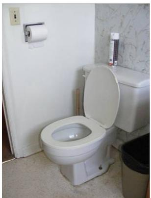
4. **Restroom is totally inaccessible due to numerous inconsistencies.** Inconsistencies include, but are not limited to, insufficient maneuvering and fixture clearances, inappropriate maneuvering space at entrance doors, no knee space at lavatory, inappropriate lavatory faucet controls, noncompliant shower, flush valve controls located on narrow side, no grab bars at water closets or
