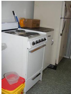
6. **Kitchen is inaccessible due to numerous inconsistencies.** UFAS requires kitchens to comply with 4.34.6. Inconsistencies include, but are not limited to, no knee space (or removable base cabinets) at sink, round controls at sink faucet, insufficient clearance at entry to kitchen (only 29"), countertops too high, no accessible work space, insufficient clearances at appliances, appliances don't meet all UFAS requirements.
