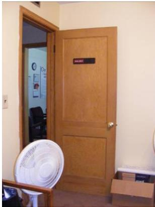
1. **Round door hardware exists on interior and exterior doors.** Doors are required to have opening hardware, which does not require tight grasping or twisting of the wrist to operate. Modify doors by replacing door knobs with lever-type hardware or installing add-on levers.
