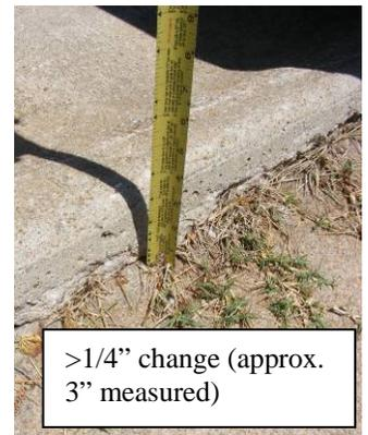
**EXISTING CONDITION: No accessible route exists connecting the parking lot with the route (sidewalk) to the office and apartments due to an abrupt change in level (curb) of approximately 3”.** According to ADAAG, changes in level up to 1/4 in (6 mm) may be vertical and without edge treatment (see Fig. 7(c)). Changes in level between 1/4 in and 1/2 in (6 mm and 13 mm) shall be beveled with a slope no greater than 1:2 (see Fig. 7(d)).
