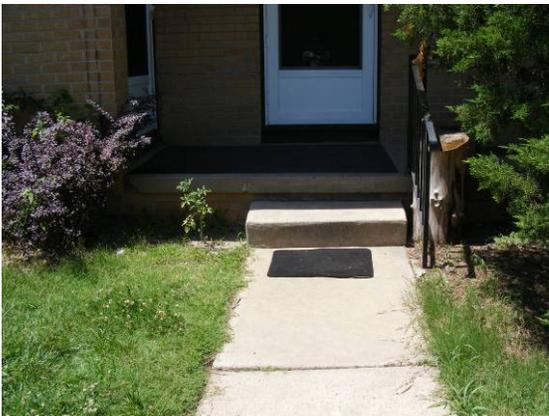
**EXISTING CONDITION:** The main public entrance consists of two doors in series with insufficient space between the two doors. According to ADAAG, the minimum space between two hinged or pivoted doors in series shall be 48 in (1220 mm) plus the width of any door swinging into the space. Doors in series shall swing either in the same direction or away from the space between the doors (see Fig. 26).
