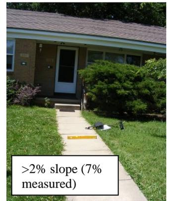
**EXISTING CONDITION:** Abrupt changes in level and steep cross slopes exists on the path of travel (sidewalk) leading to the apartments and the office. According to ADAAG, changes in level up to 1/4 in (6 mm) may be vertical and without edge treatment (see Fig. 7(c)). Changes in level between 1/4 in and 1/2 in (6 mm and 13 mm) shall be beveled with a slope no greater than 1:2 (see Fig. 7(d)). According to ADAAG, nowhere shall the cross slope of an accessible route exceed 1:50 (2%).
