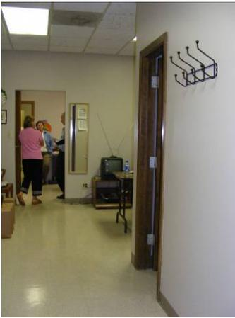
**EXISTING CONDITION:** Coat rack is located too high at 5'-7" and creates a protruding object by projecting 4-3/4" from the wall.
