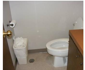
**EXISTING CONDITION:** Round door opening hardware exists on many interior and exterior doors within the employee work area. According to ADAAG, accessible doors are required to have opening hardware, which does not require tight grasping or twisting of the wrist to operate.
