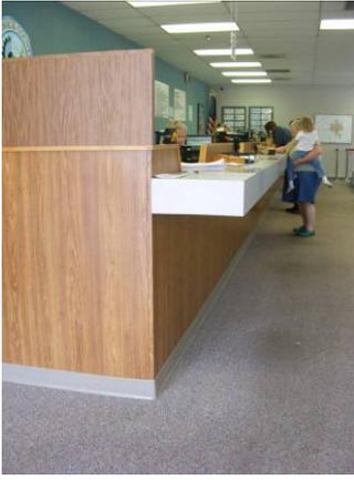
**EXISTING CONDITION:** Transaction counter creates a protruding object in the public area. Where objects protrude from walls more than 4-inches and their leading edge is higher than 27-inches and lower than 80-inches, these objects are considered protruding objects, which may not be detectable by individuals who are blind and use a cane.
