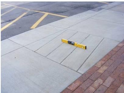
**EXISTING CONDITION:** The curb ramp, connecting the street (parking lot) level with the sidewalk level, does not provide an appropriate detectable warning surface. The existing curb cut has a detectable warning surface. However, this detectable warning does not comply with current ADAAG specifications regarding truncated domes.
