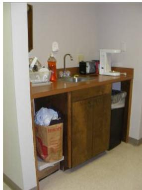
**EXISTING CONDITION:** Sink is too high, does not provide appropriate knee clearance due to cabinets underneath, and has round knob for faucet controls.
