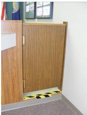
*It should also be mentioned that doors (or gates) at the same location as a step (with no landing), create a safety hazard and generally are not allowed by the building code.*
