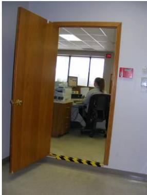
*It should also be mentioned that doors at the same location as a step (with no landing), create a safety hazard and generally are not allowed by the building code.*
