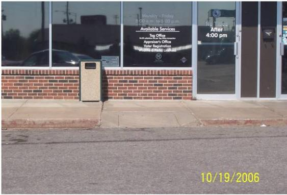
**EXISTING CONDITION:** The curb ramp east of the main entrance, connecting the street (parking lot) level with the sidewalk level, does not provide an appropriate detectable warning surface and has very steep side flares (as identified in Kent Johnson’s November 2006 report).
