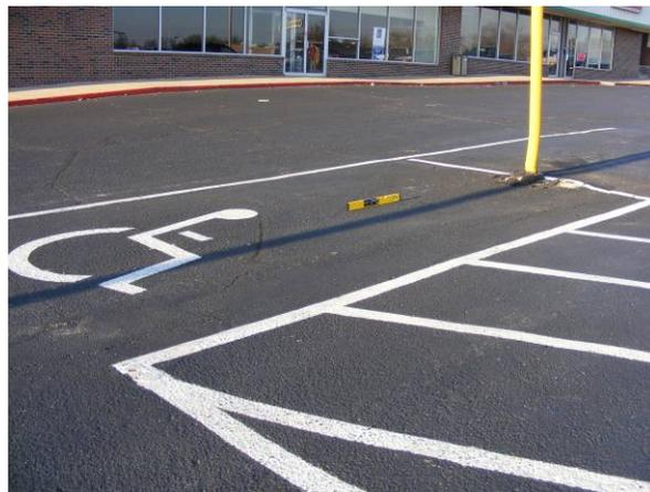
**EXISTING CONDITION:** Accessible parking spaces west of main entrance exceed allowable slope as shown above. Existing slopes measured over 4%.
