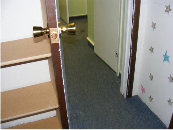
**EXISTING CONDITION: Round hardware exists on interior doors; doors have less than 32” clear opening.**
