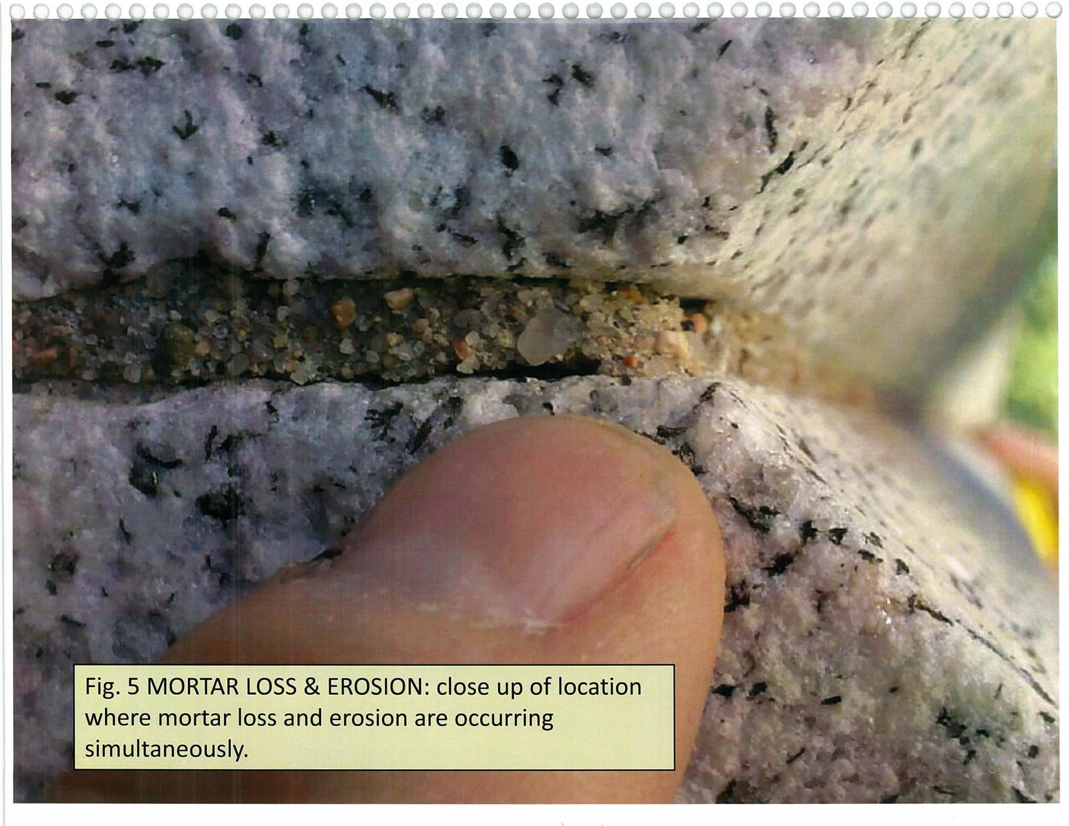
Fig. 5 MORTAR LOSS & EROSION: close up of location where mortar loss and erosion are occurring simultaneously.
