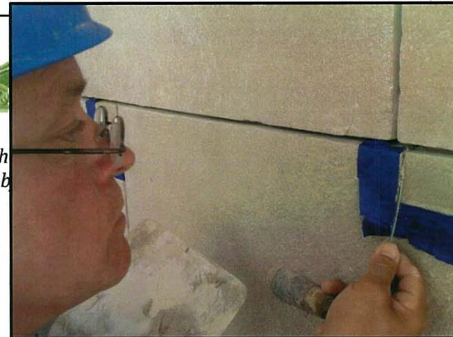
**Fig.12 Project Award & Onsite SPC Historic Masonry Training:** Individual proficiency skill training for each mason at the project site. Training certificates earned by the individual mason and not by the company. Each mason must pass a written test and demonstrate proficiency of intended learning outcomes by installing a test panel. The test panel must be reviewed and approved by a project peer review committee in order to receive a certificate and hard hat sticker shown left bottom.
