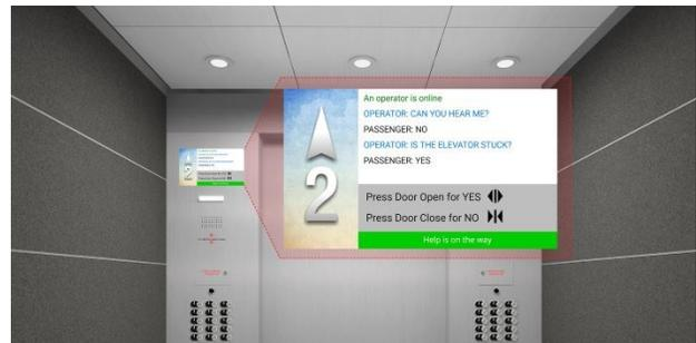
ASME A17.1 Chapter 2 Section 2.27.1.1.3—The code also requires a means to display video to observe passengers at any location on the car floor, to authorized personnel for entrapment assessment.
