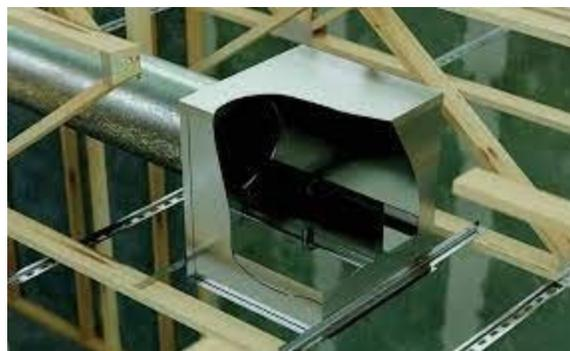
**607.6.2.1.2 Static systems.** Static ceiling radiation dampers shall be installed only in systems that are not designed to operate during a fire. Exceptions:
