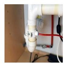
The air gap faucet meets the code requirements to prevent the potential cross connection of a direct connection between the RO system and the drainage system. The non-air gap single tube faucet does not meet the code requirements and is considered an unlawful connection. All that money and effort to provide clean water just to be cross connected right there under the sink. SMH (shaking my head).
